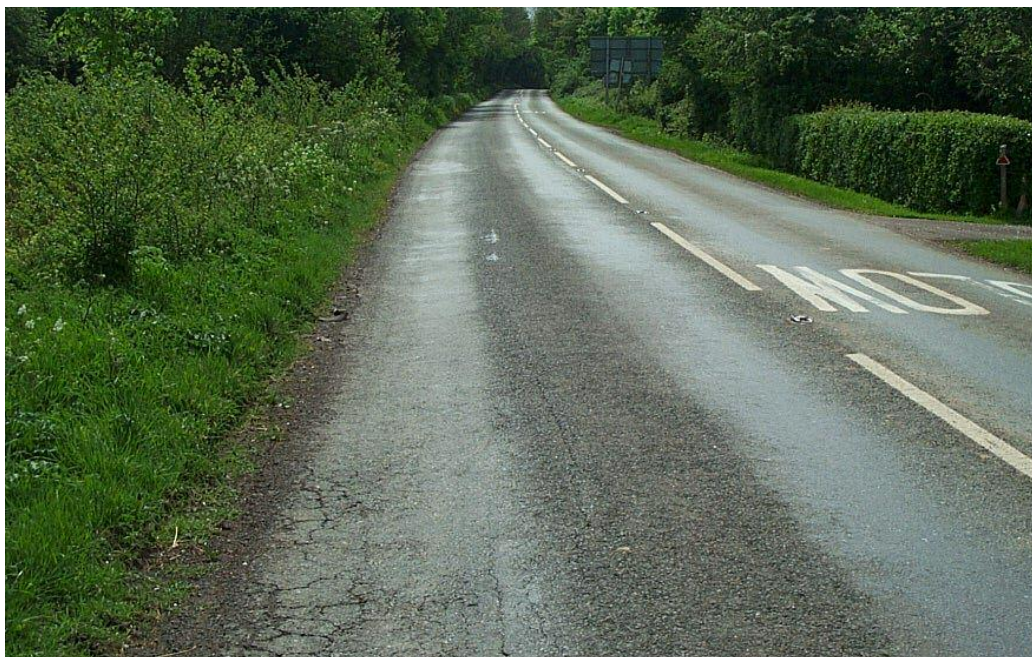
Figure 2.7 Variation in average texture depth across the road surface
