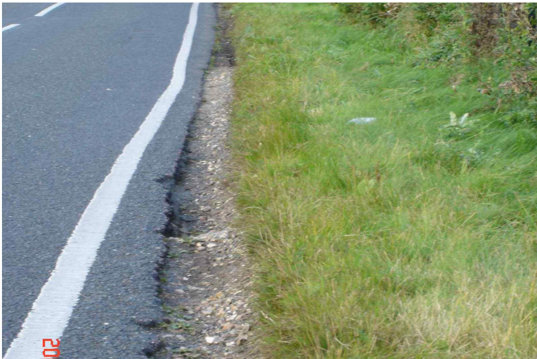
Figure 2.5 Examples of edge steps LES1 and LES2 identified by SCANNER on a minor road
